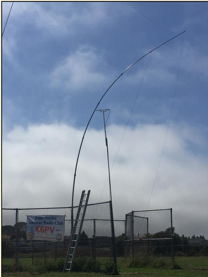
**Oops:** Fiberglass mast for K6PV 160-meter antenna starts to bend before being corrected. This year was our first-ever attempt using 160-meters during Field Day but we heard no other stations. PHOTO: MALIN DOLLINGER, KO6MD
