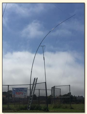
**Oops:** Fiberglass mast for K6PV 160-meter antenna starts to bend before being corrected. This year was our first-ever attempt using 160-meters during Field Day but we heard no other stations. PHOTO: MALIN DOLLINGER, K06MD
